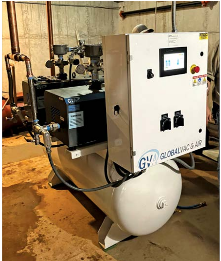
The duplex vacuum pump system was bolted together onsite.
