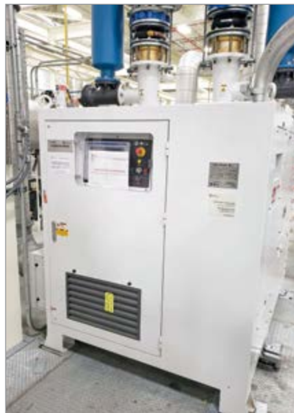
The turbo aeration blowers in these pictures were installed for a major paper consumer goods manufacturer in 2019.
