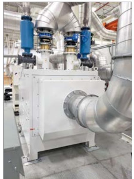
The turbo aeration blowers in these pictures were installed for a major paper consumer goods manufacturer in 2019.
