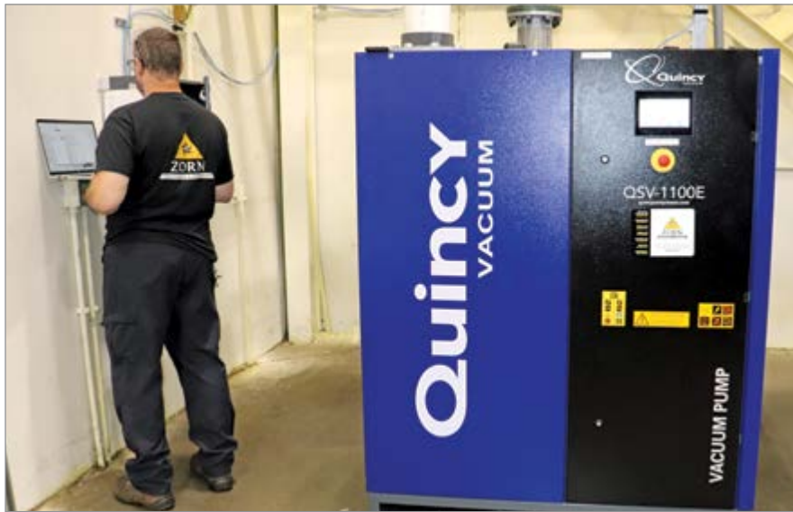
The vacuum system audit showed one 50 hp VSD vacuum pump was able to do the work of three older model 40 hp fixed-speed vacuum pumps.
