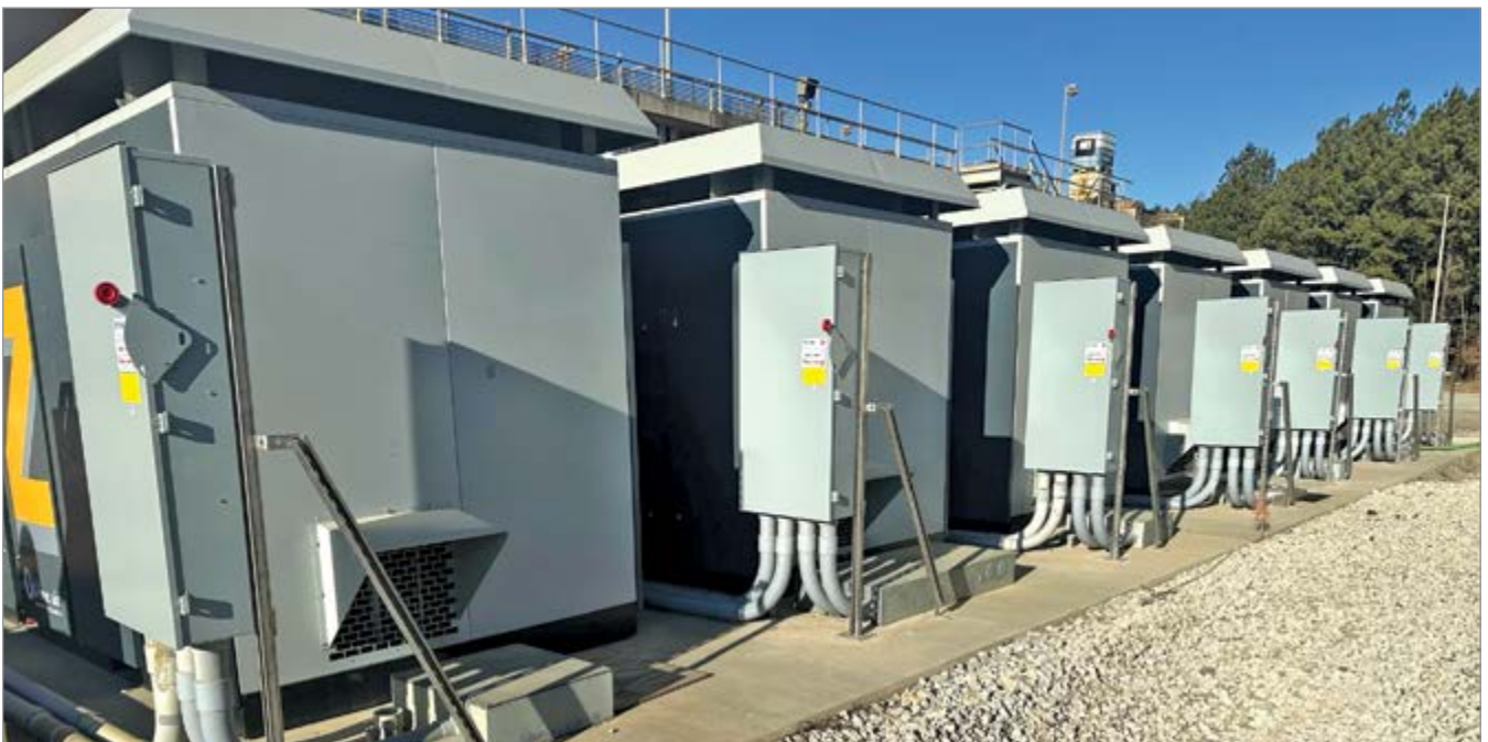
The completed installation of an aeration blower system
