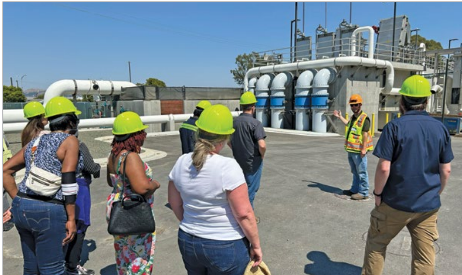
Veolia North America invested $40 million for upgrades to the Richmond Water Pollution Control Plant.
