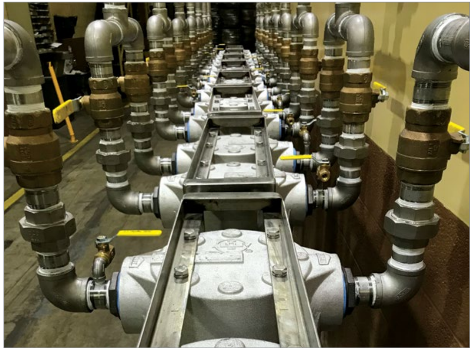
This inventory of duplex vacuum filters allows the user to maximize uptime and offers exceptional flexibility for a manufacturing process.
